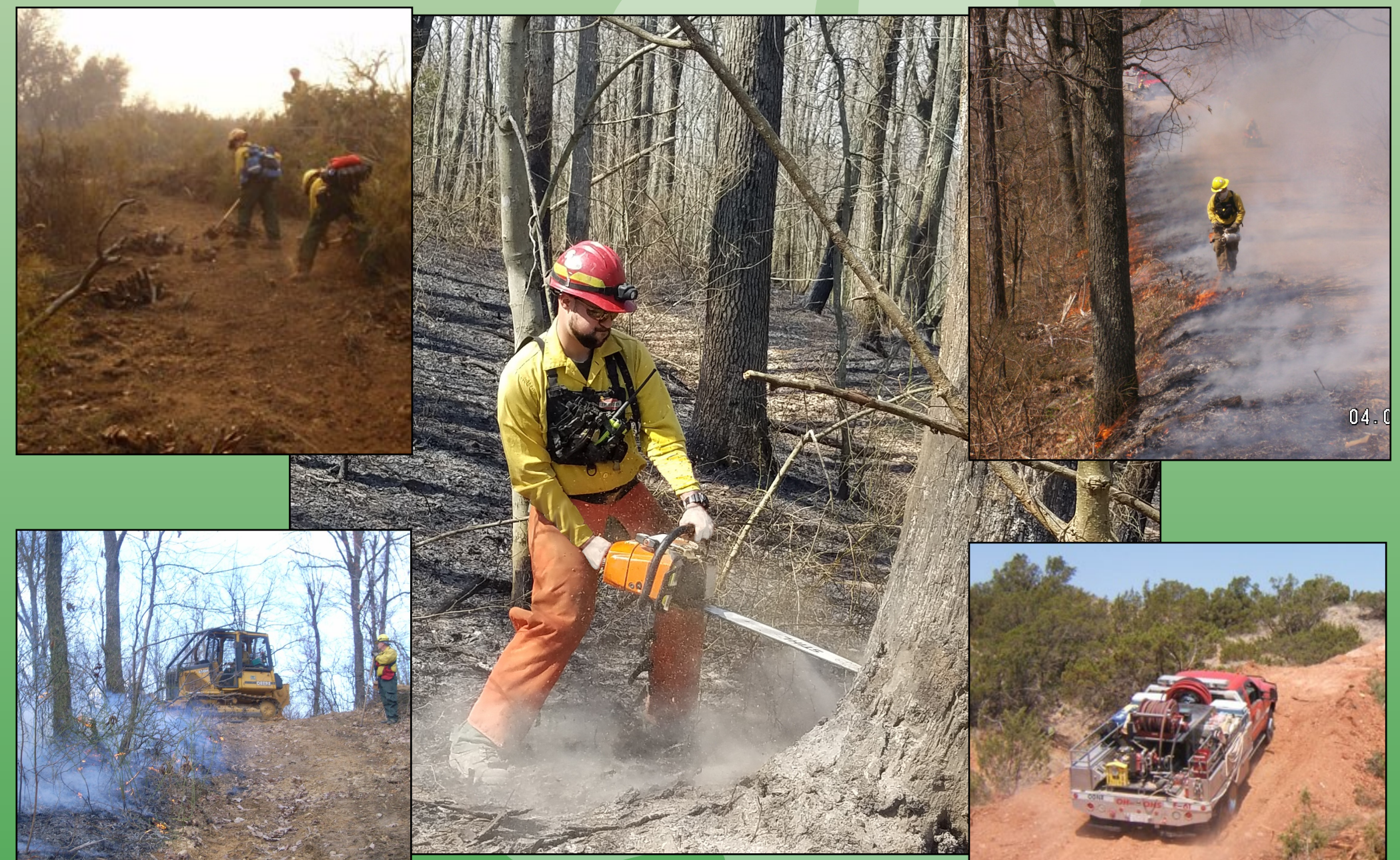
Fire fighting tools. Hand tools such as fire rakes and Pulaski axes ( top left ), leaf blowers, and bulldozers ( bottom left ) are used to remove fuels down to bare soil. Chainsaws ( center ) are used to remove large fuels and take down dead burning trees. Fire ( top right ) can be used to burn off fuels to stop fire spread. When possible, engines with water pumps ( bottom right ) can be used to control fire and eliminate smoldering fuels.
